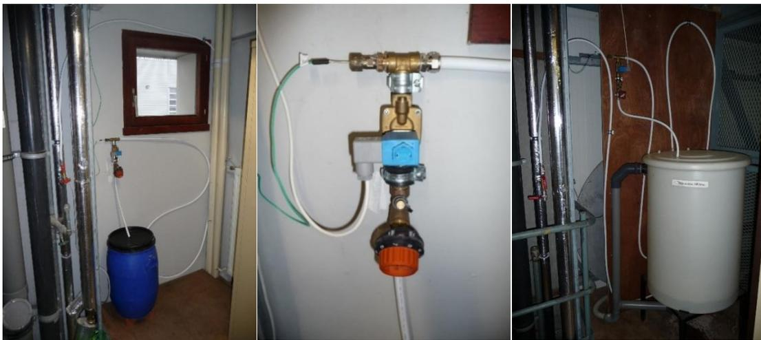
**Figure 5 - views of the 'kitchen' draw-off (on the left); the 'shower' draw-off (center) and their equipments : temperature probe; electro valve and regulating valve at the reservoir connections (on the right).**
